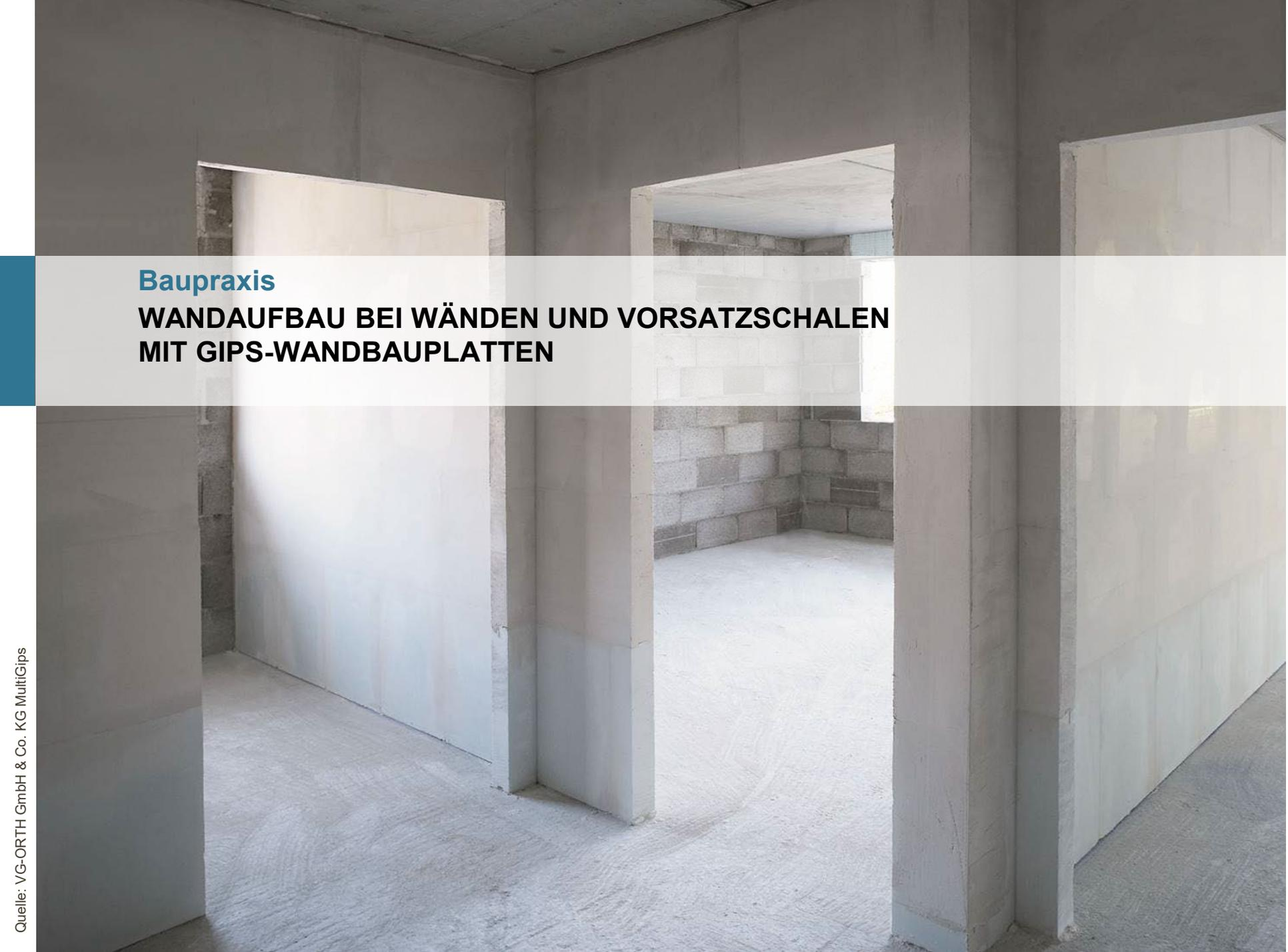
The image shows the interior of a room during construction. The walls are primarily composed of light-colored gypsum boards (Gips-Wandbauplatten) mounted on a concrete frame. In the background, a room is visible where the walls are made of grey concrete blocks (Vorsatzschalen). The floor is a smooth, light-colored concrete surface. The lighting is bright, likely from a window or door in the background room.
