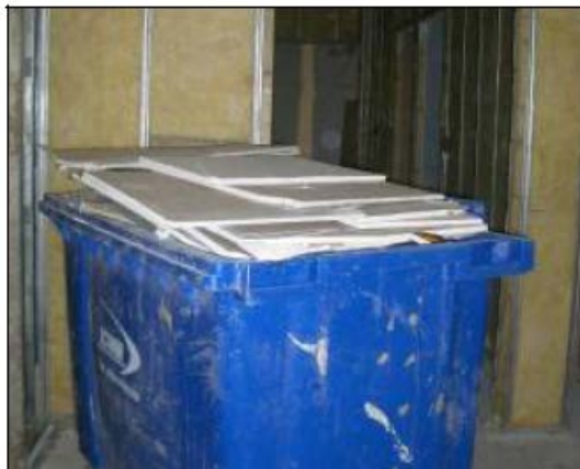
660 litre wheelie bin containing plasterboard waste
