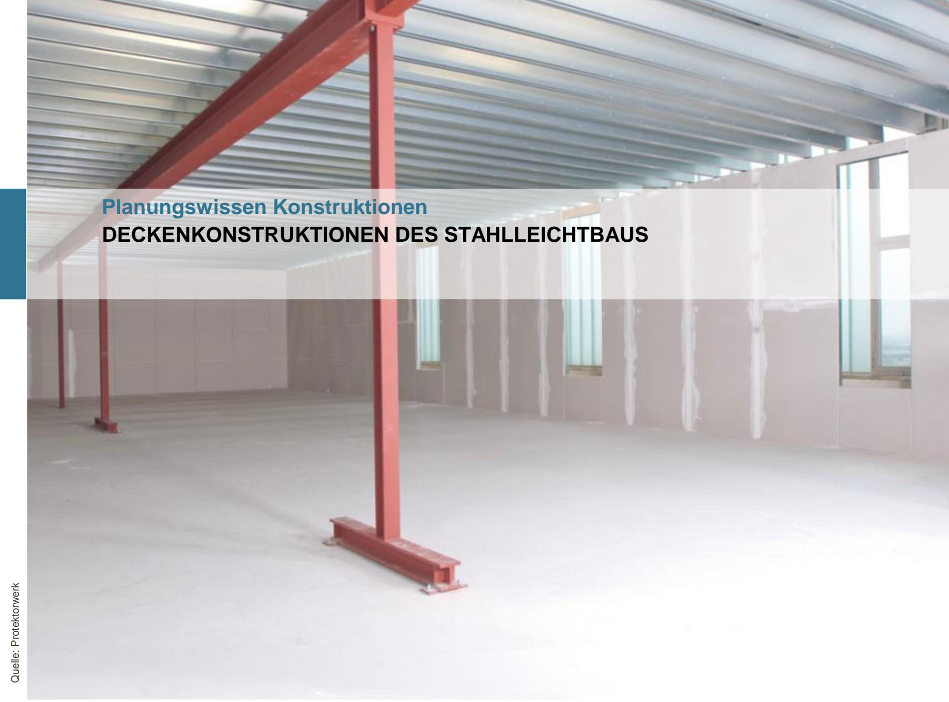
The image shows the interior of a building under construction. The structure is a steel frame with red-painted steel columns and beams. The ceiling consists of a grid of steel joists with corrugated metal decking. The walls are partially finished with light-colored panels, and there are several windows. A semi-transparent text box is overlaid on the upper part of the image.
